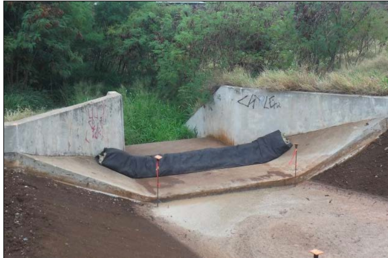
Image Source: State of Hawaii Department of Transportation, Highways Division, Construction Best Management Practices Field Manual , 2021.
